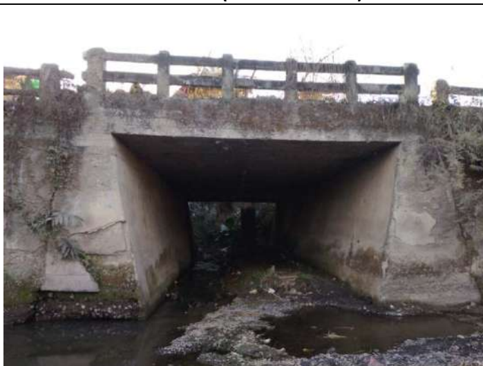
RCC Slab Bridge (Ch. 2.380 Km)
