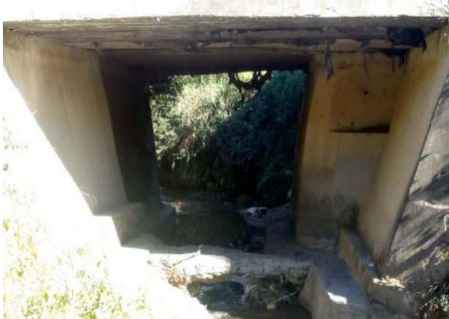
RCC Slab Bridge (Ch. 6.932 Km)
