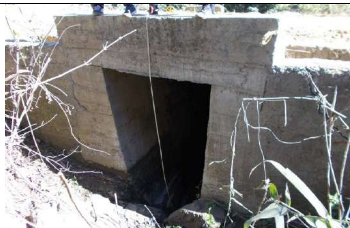
Slab Culvert (Ch. 44.482 Km)
