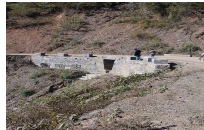
Slab Culvert (Ch. 35.494 Km)
